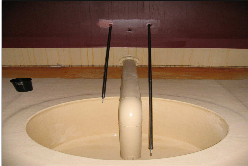
Fig. 4. View of the sump, control probe and alarm probe
