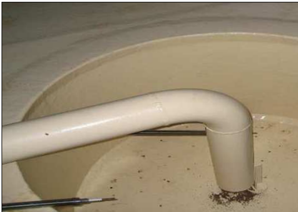
Fig. 3. View of the sump and the control probe
